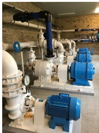
Figur 6: Rentvandspumper
